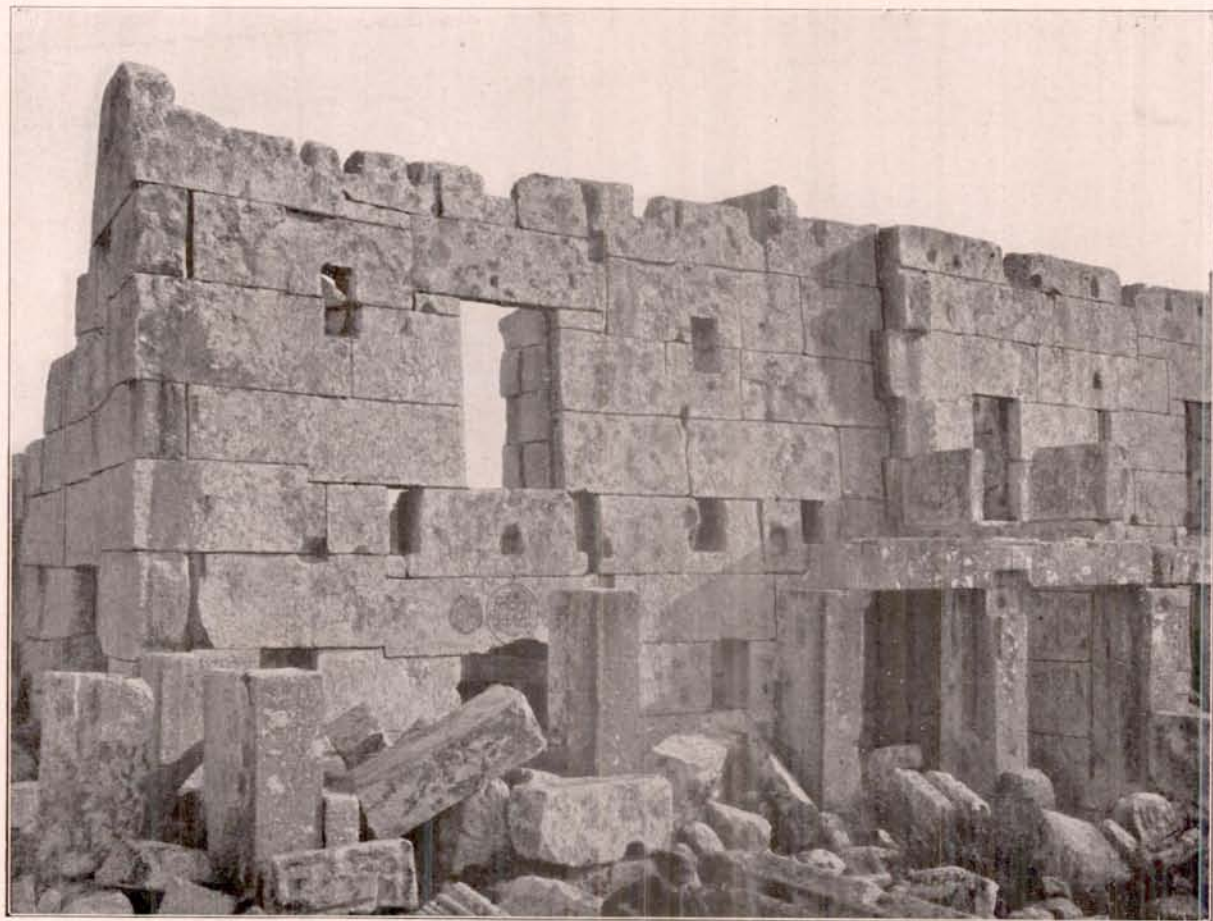
Ill. 327. Kefr Nabū. Inn, West End. View from the Southwest.
