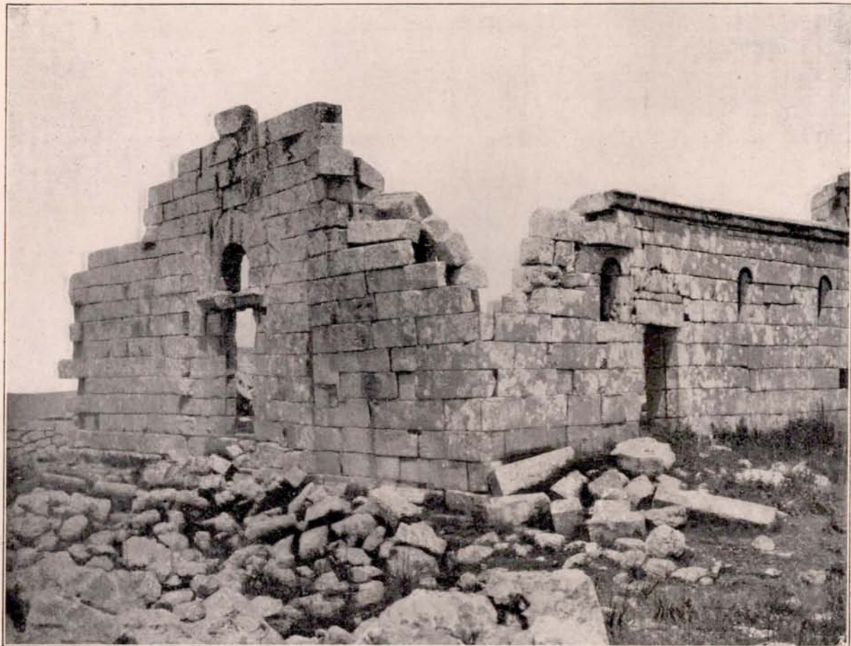
Ill. 356. Qal'at Kalôtâ; Temple-Church. View from the Southwest.
