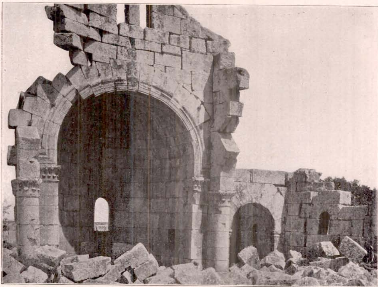
Ill. 351. Kalôtiā; East Church, Interior. View looking Southeast.
