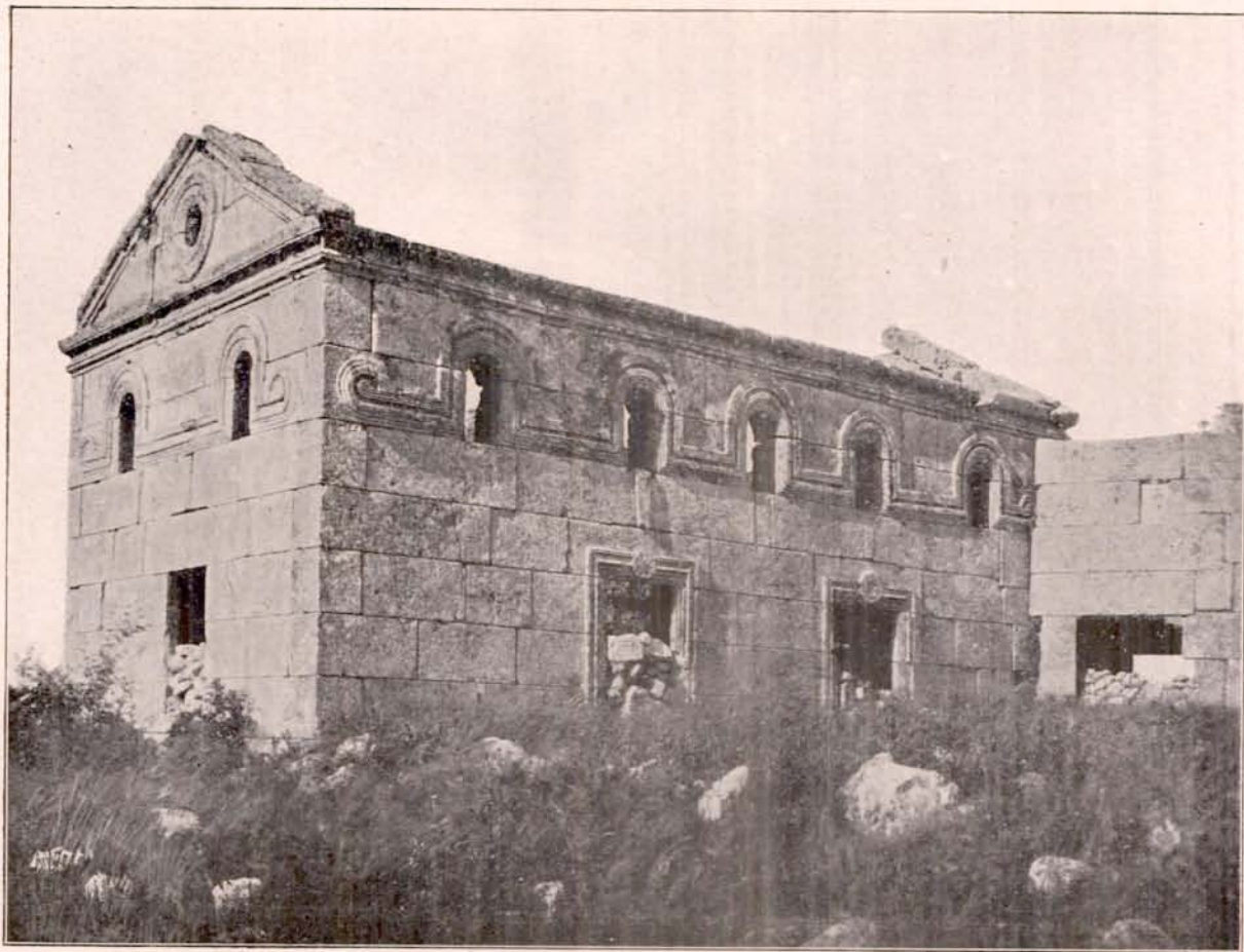
Ill. 316. Burdj Hédar; Chapel. View from the Southwest.
