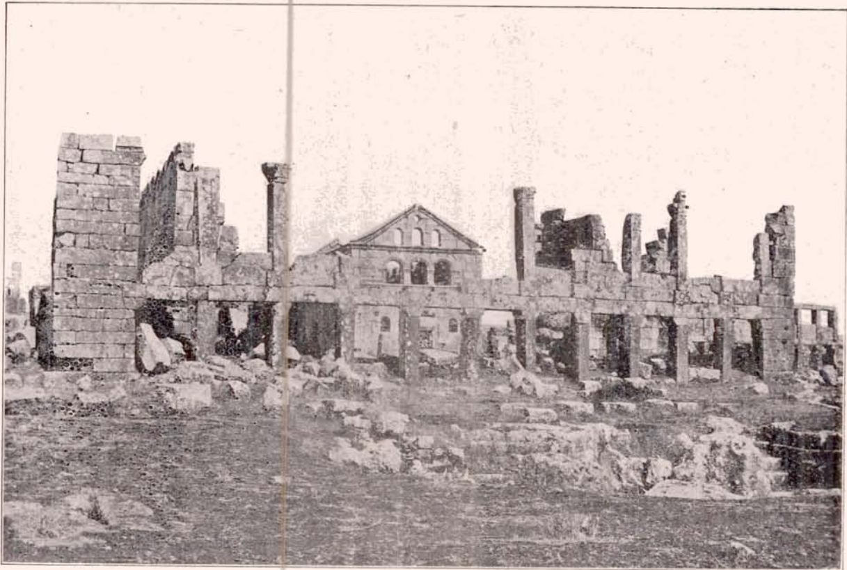
Ill. 282. Dêr Sim'ân; South Monastery. View from the West.
