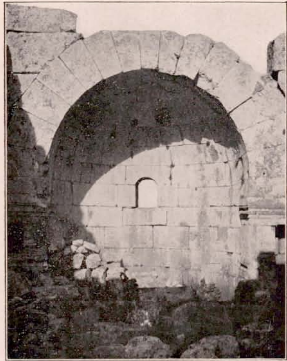
Ill. 361. Kharâb Shems; Chapel, Interior of Apse.
