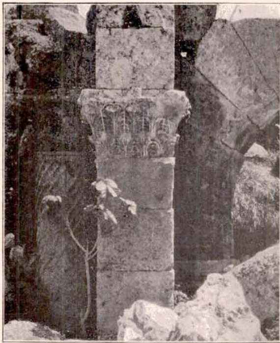
Ill. 305. Başufân; Church of St. Phocas, Column of Apse, Pier-cap and Arch of Prothesis.
