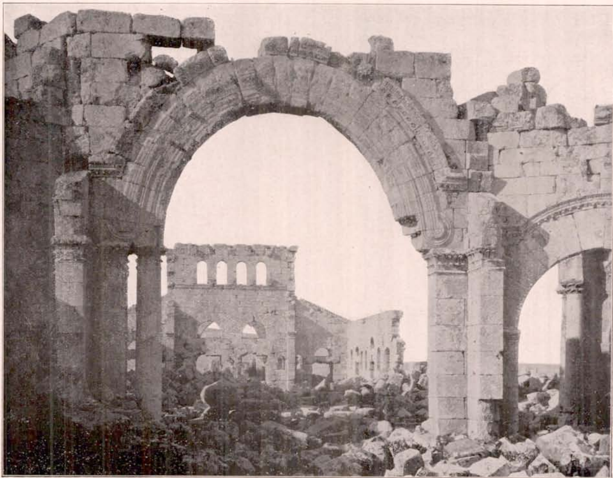
Ill. 303. Qal'at Sim'an; Northern Arch of Octagon, from the inside. View looking South.
