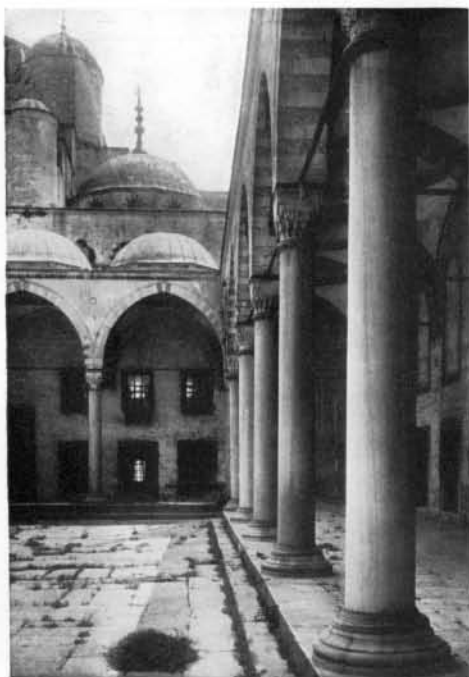
Fig. 28. Courtyard of the Mosque of Ahmet
