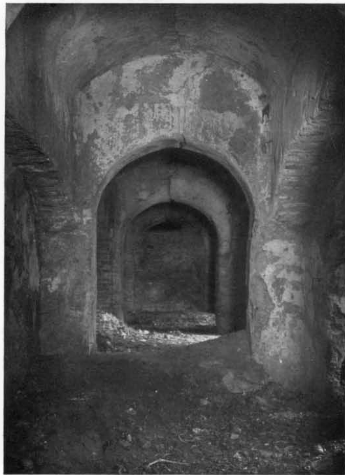
Fig. 22. Main corridor along the side
