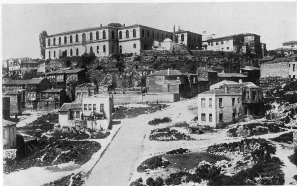
Fig. 19. The exterior of the Sphendone
