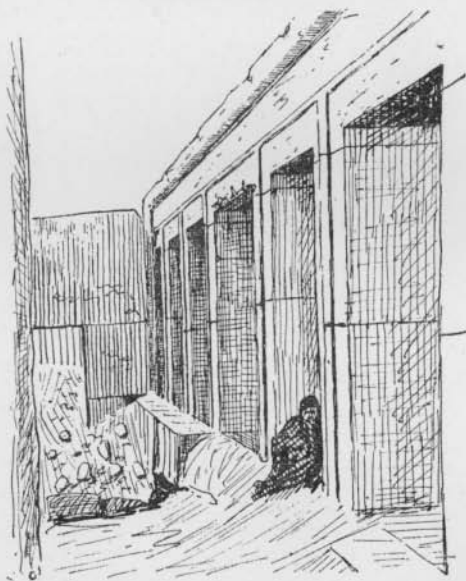
79. INTERIOR OF BUILDING.
