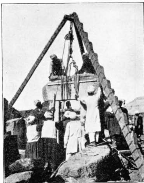
FIG. 11.—RE-ERECTION OF A FALLEN LINTEL IN THE HAREM
