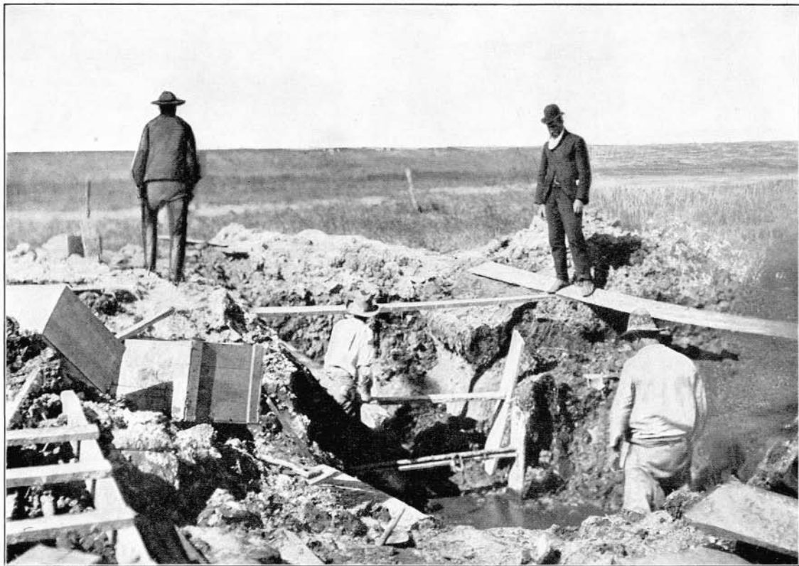
DIFFICULTIES MET WITH IN MAKING EXCAVATIONS.
