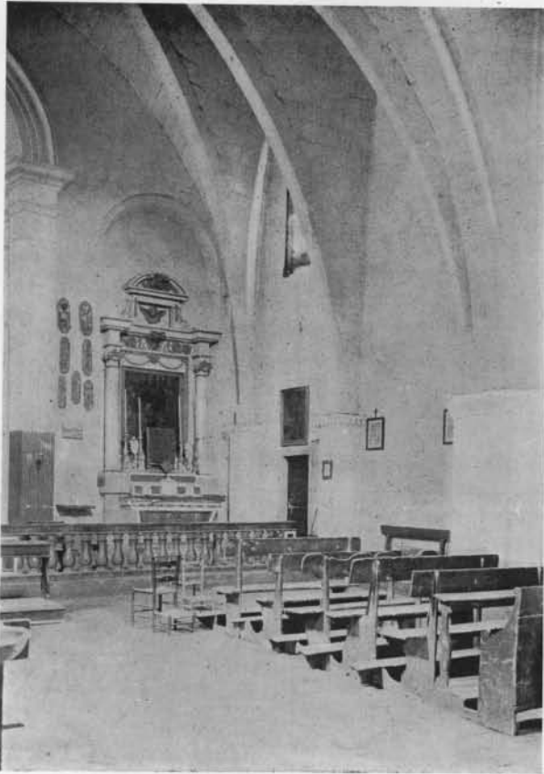
Fig. 5. The rib vault in Italy, built without solid centering. Sexpartite vault in S. Pancrazio, Corneto-Tarquiniæ. Dating about 1160.
