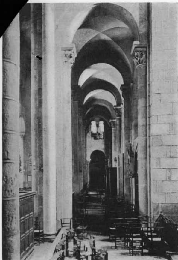
Fig. 7. The groin cross-vault in France. Built with solid centering. North aisle Notre-Dame-du Port, Clermont-Ferrand (Puy-de-Dôme). Dating twelfth century.
