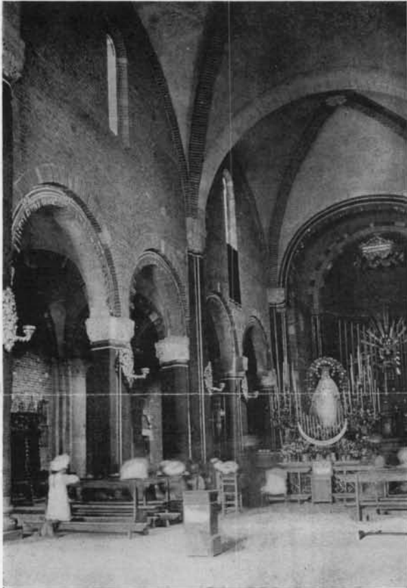
Fig. 6. The rib cross vault in the nave, associated with groin vaults in the aisles, both built without solid centering. S. Savino, Piacenza. Consecrated in 1107. Naves were not rib-vaulted in the Ile-de-France until 1125.
