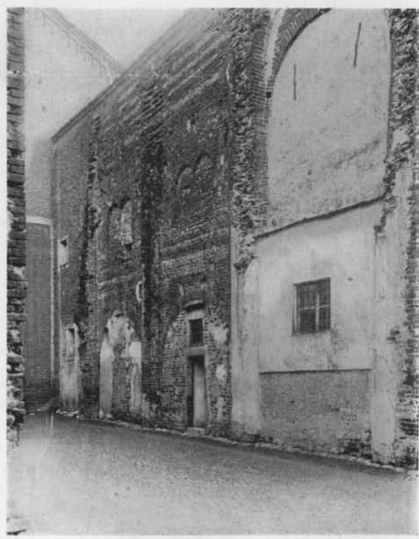
Fig. 4. Church of San Nazaro at Sannazaro Sesia (Province of Novara). Ruined interior of the nave, showing compound piers, with shafts which supported a rib vault built without solid centering. Dating 1040. This is eighty-five years earlier than the first rib-vaulted nave in the Ile de France.
