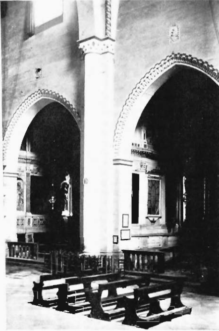
FIG. 16. THE CATHEDRAL, VICENZA. From a Survey photograph of 1901. Showing the depth of the chapel walls.
