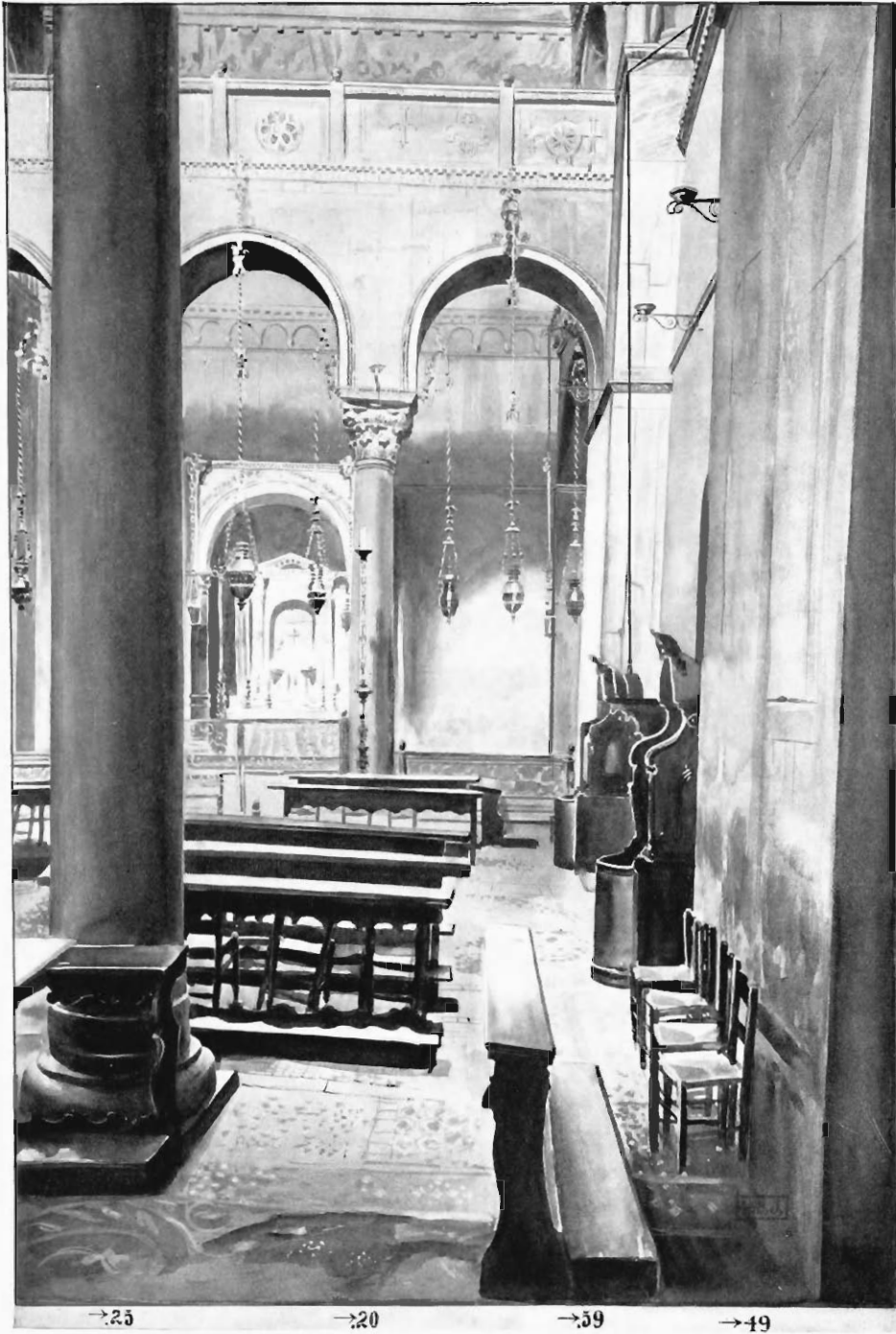
FIG. 33. ST. MARK'S. SOUTH TRANSEPT, LOOKING EAST.
