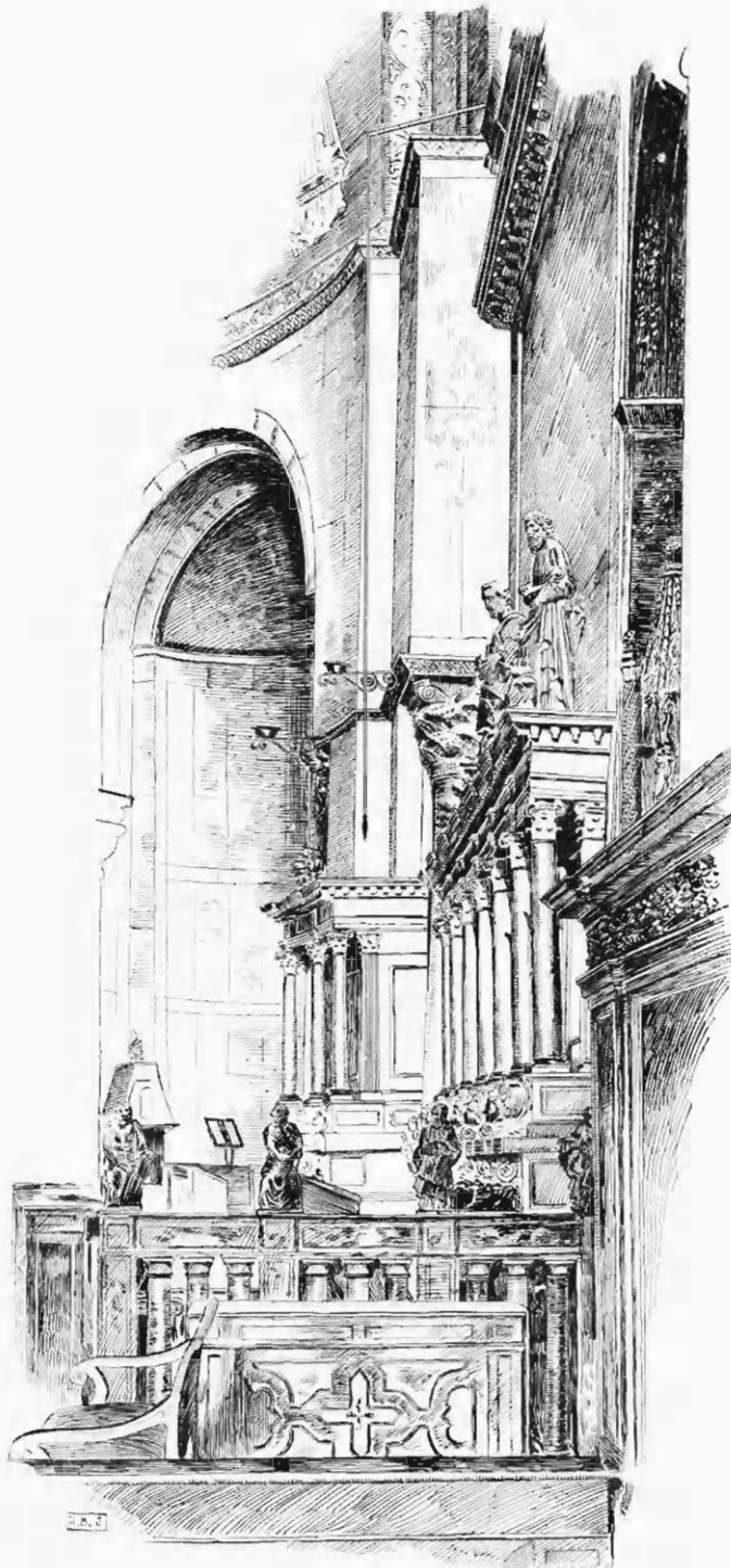
FIG. 40. ST. MARK'S. VIEW OF THE APSE.
