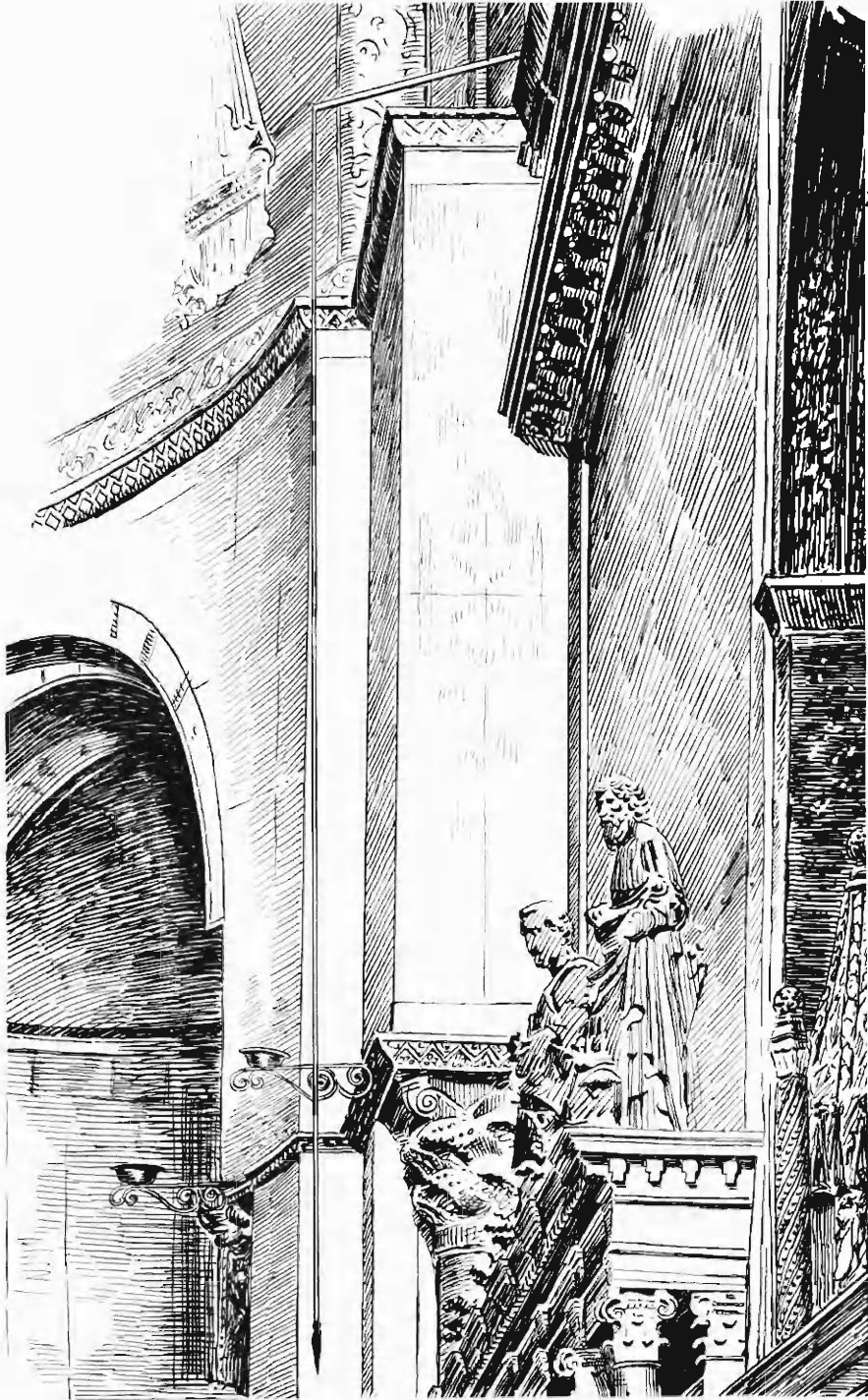
FIG. 41. ST. MARK'S. PLUMBING THE APSE.
