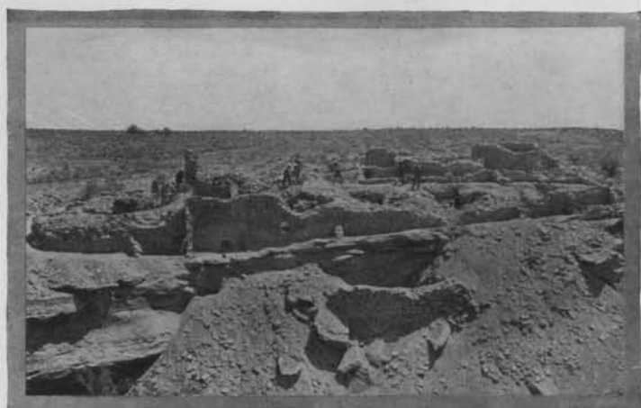
EXCAVATION WORK ON COMMUNITY HOUSE
