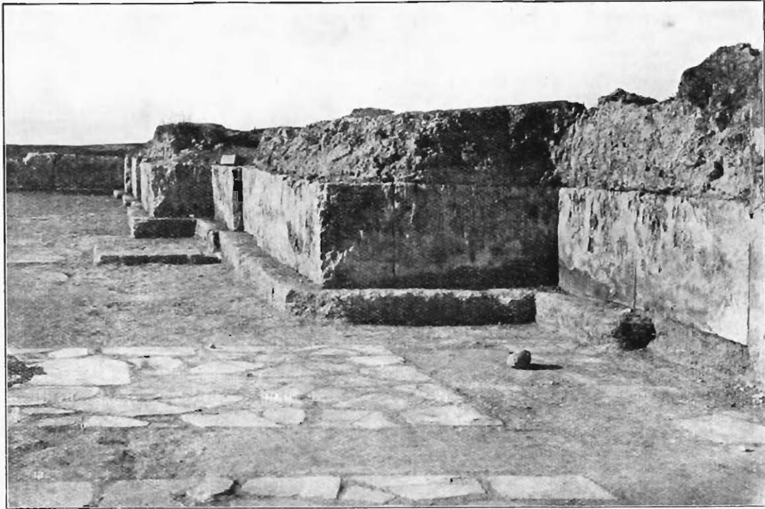
View of Part of West Wall of Palace, Knossos, from West Porch.
