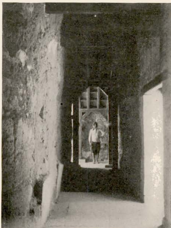
FIG. 16.—VIEW IN LOWER EAST-WEST CORRIDOR (LOOKING E.).
